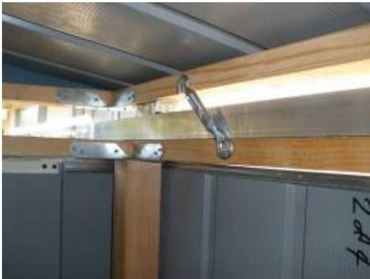
*Turnbuckles keep the roof in place*
